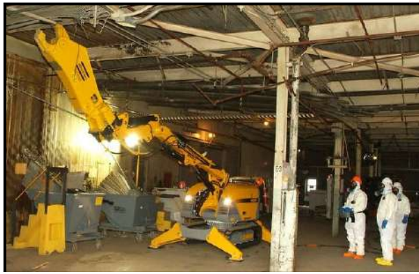
Figure 47:- Robot Demolition
