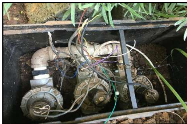
Fig. 53:- Poor quality cabling
