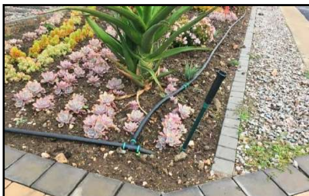
Fig. 50:- Inadequate trenching
