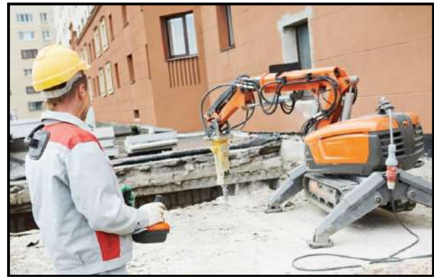
Figure 47:- Robot Demolition
