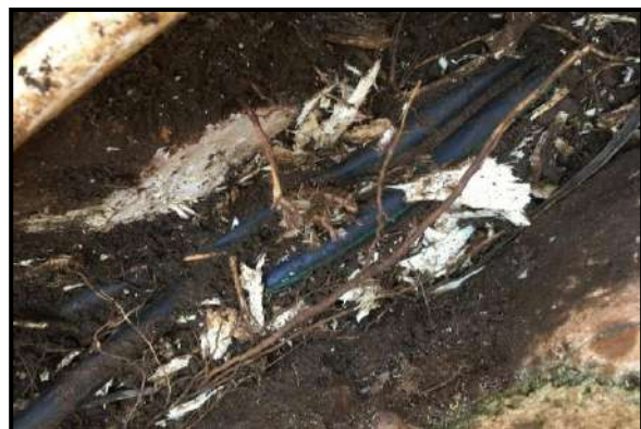
Fig. 55:- Pipes crimped by tree roots
