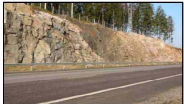
Rock Face Cutting (Shielded with Safety Barrier)
