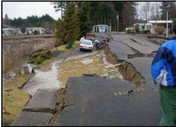
Fig. 24:- Soil Liquefaction on road
